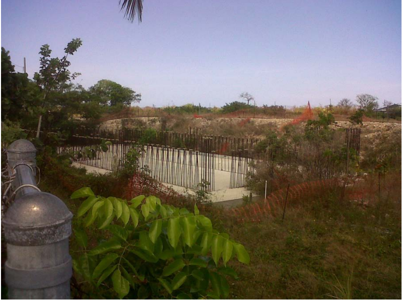
Exhibit 11: Beulah Smith High School building site, March 2012
