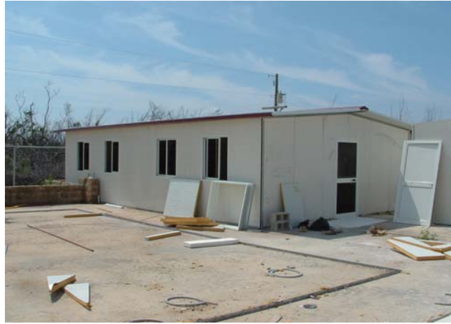
Unit substantially completed externally
